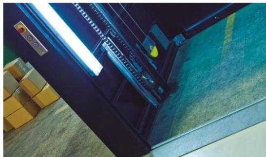
The freestanding modular structure incorporates a 100mm shaft pit, requiring a straight-forward loading ramp. As an alternative, a 100mm pit can be built below the structure.
